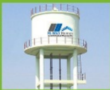
Overhead Water Tank
